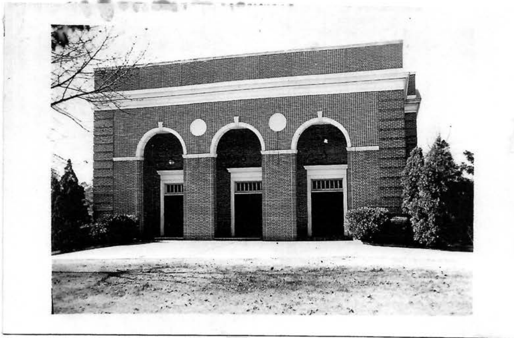
New City Auditorium, East Point, Georgia.
